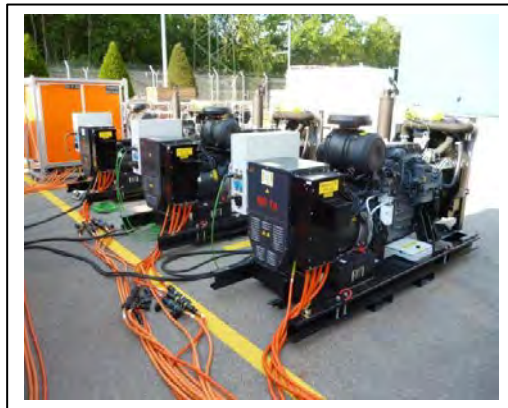
Figure 5: Testing of mobile emergency power generators.
