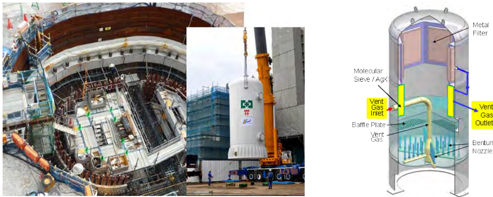
Figure 12: Installation of Filtered containment venting systems (FCVS) [11].
