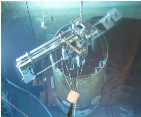
Figure 3: Underwater cut of the upper internal
