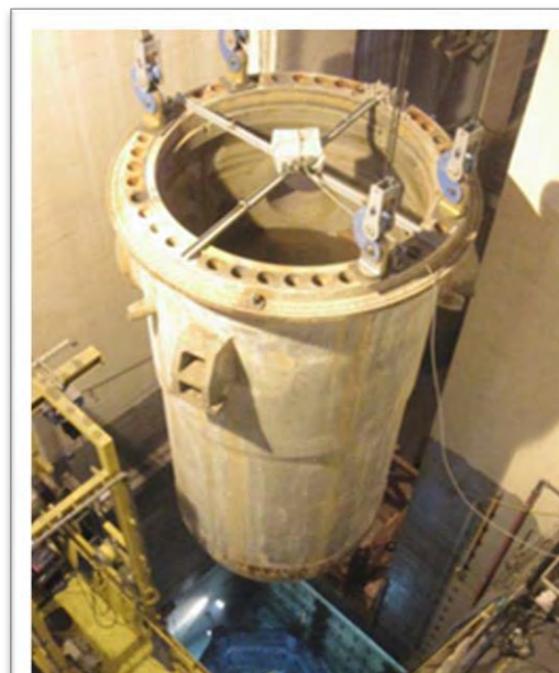
Figure 2: Transfer of the reactor vessel
