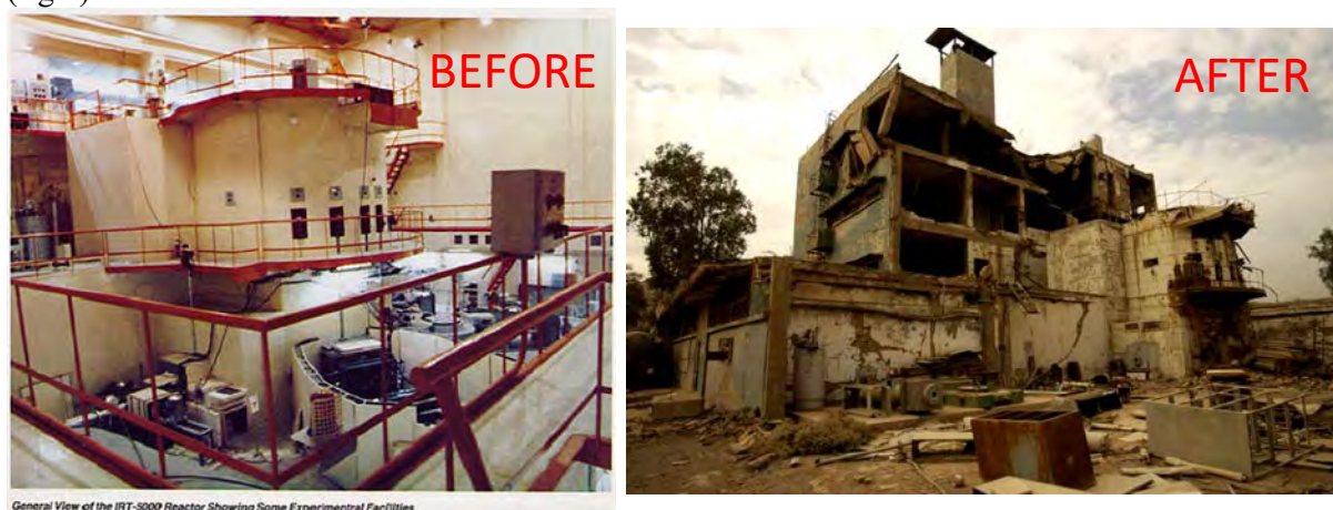
Figure 1: Iraq's IRT-5000 research reactor during operation (left) and after being bombed in 1991 (right).
