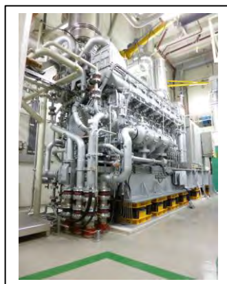
Figure 4: Emergency diesel on new aseismic bumpers.
