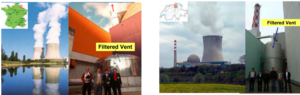
Fig. 9 Filtered containment venting systems in Chooz NPP (PWR), France and in Leibstadt NPP (BWR), Switzerland [8].
