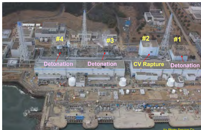
Figure 4: H 2 detonations occurred after vent operations (Units 1, 3 and 4) [11].
