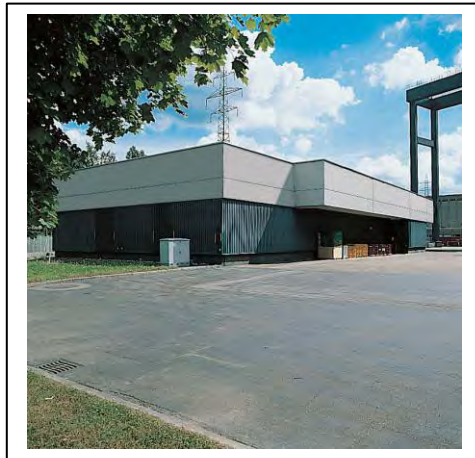
Figure 1: Bunkered emergency system building of the Goesgen NPP.
