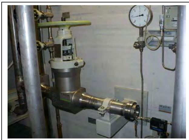
Figure 3: Fire hose fitting for steam generator water supply.
