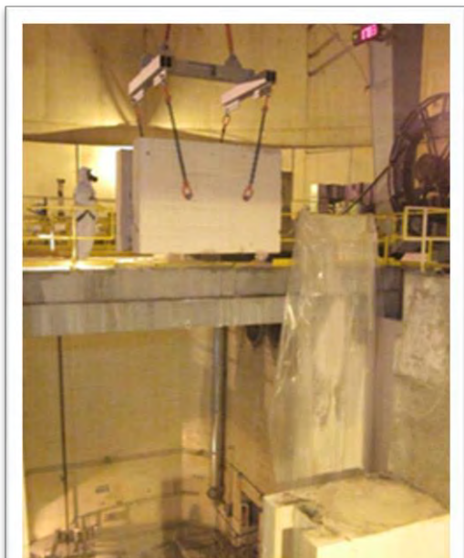
Figure 1: Cut and transfer of contaminated walls
